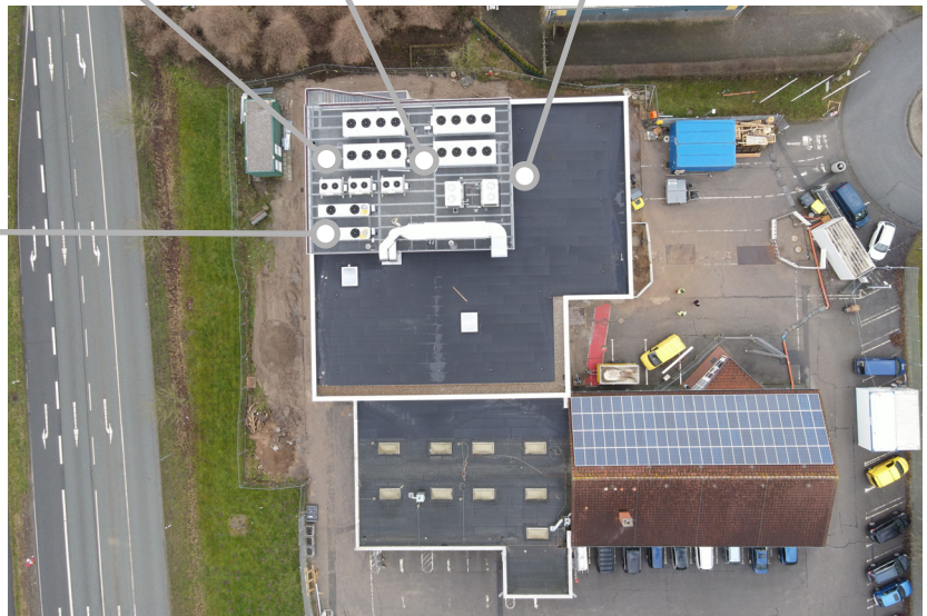
Construction of the laboratory in Harrislee, Schleswig-Holstein
