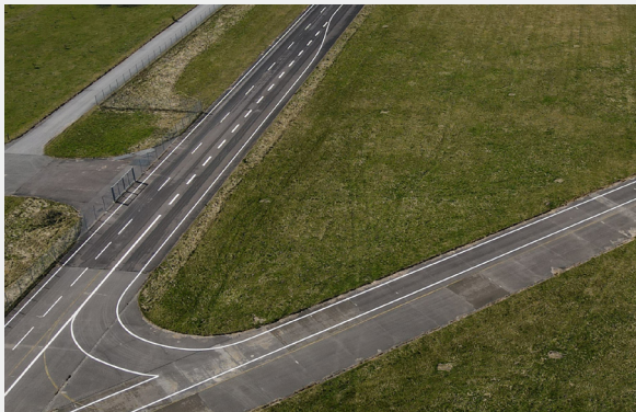
Road marking of the freeway section of the test track located in Leck (Source: KBA)
