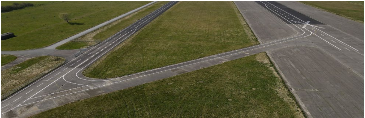
Drive up at TeCeL for test purposes
